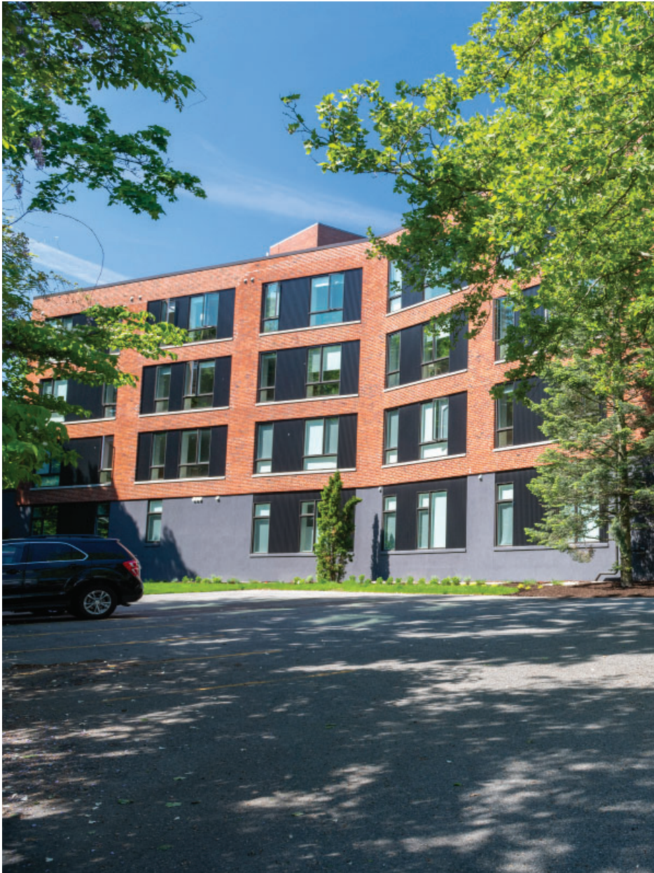
101 HILLSIDE EAST SIDE, PROVIDENCE RI RENOVATION - 22 UNITS
